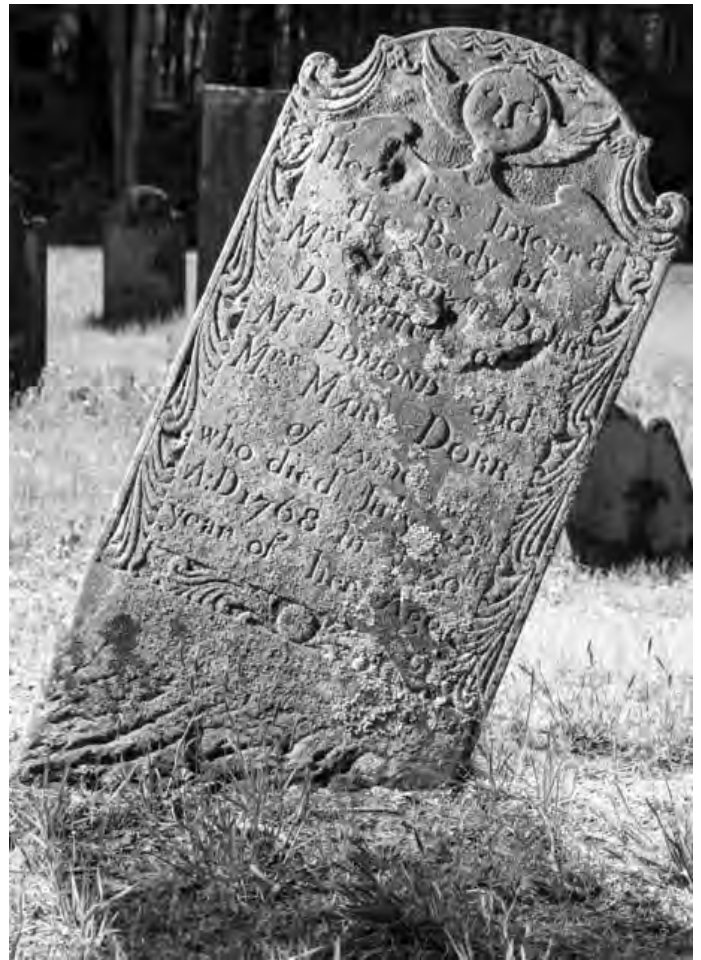
Headstones in Lyme cemeteries made from porous local sandstone are deteriorating rapidly. The carving on Deborah Dorr's stone is only partially visible.
