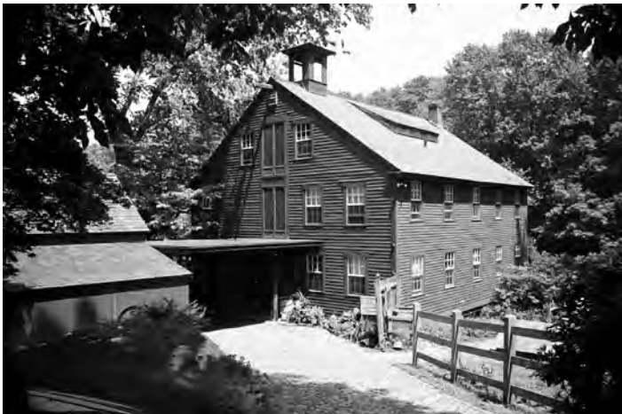
Typical architectural features of old mill buildings can be seen in the “Red Mill” (1784), on the Eight Mile River, now a residence: multi-storey with large open work spaces (for grain milling, sawing, spinning or weaving), exterior hoist to storage lofts for raw material or finished goods, and the bell to announce the working hours.
